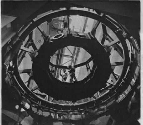
PBFA's center is the reaction chamber where high-intensity beams are focused on tiny (smaller than a toy marble) fuel pellets of deuterium and tritium.
